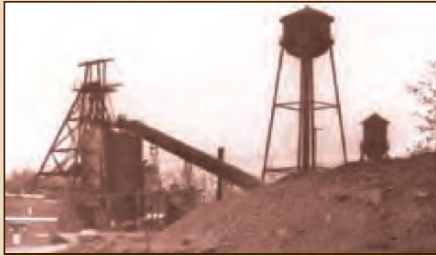
Headframe, buildings and water tanks from the Iron Mountain mine, which began mining in 1836.
